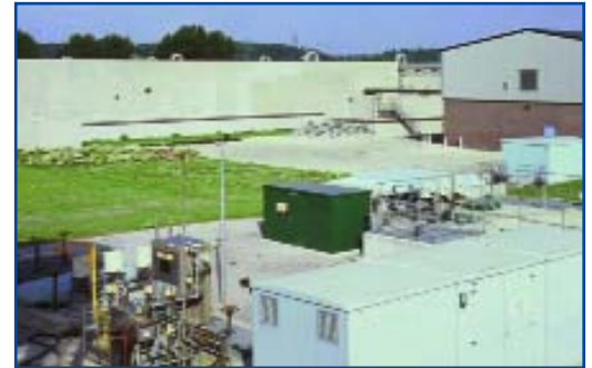
The Secondary Treatment Plant at Wessex Water's Avonmouth site.
