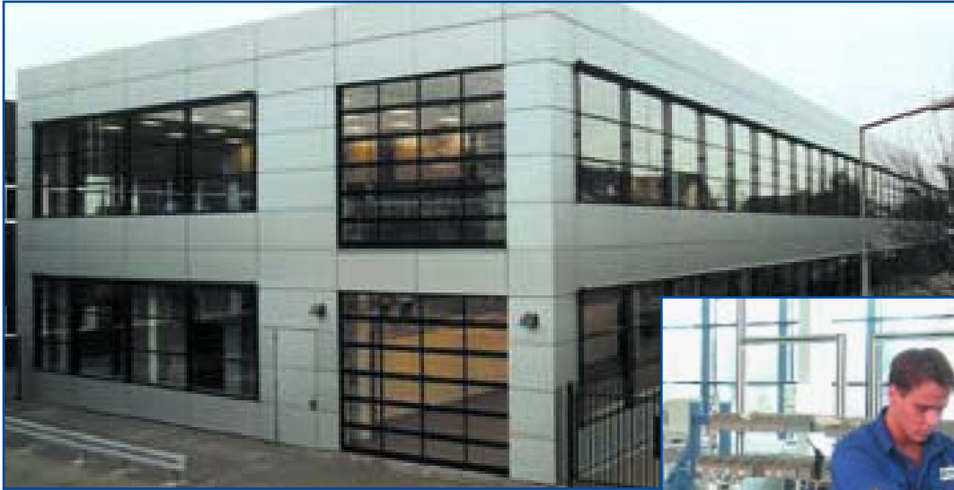
LEFT. New purpose-built filter element facility.
