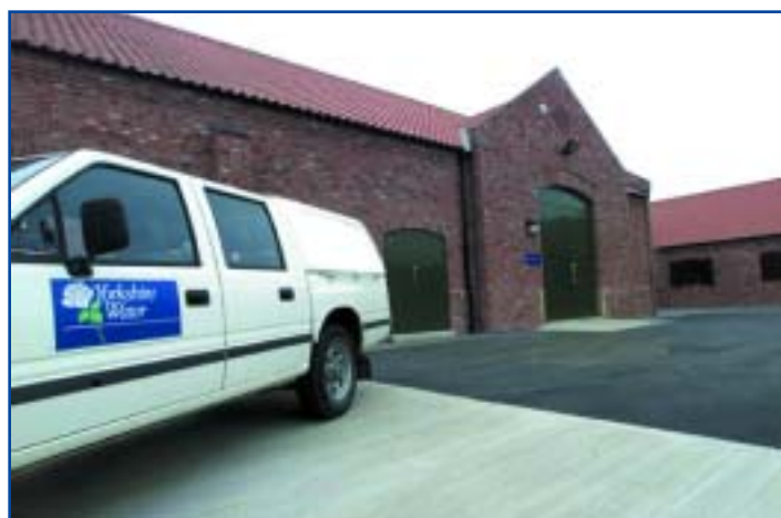
LEFT. Yorkshire Water's Keldgate site is built in the style of a farm to blend with the landscape.
